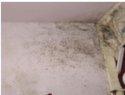
Fig. 2: Mould formation on walls and ceiling as result of poor thermal insulation and ventilation.
