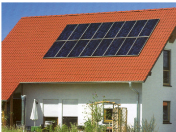
Fig. 4: Roof-mounted solar cells.
